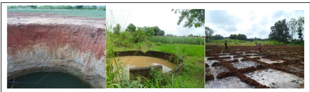
Figure 2: Agro-well construction and land development
